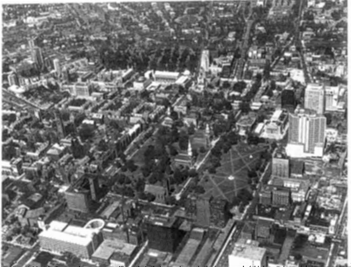
New Haven's historic Green, where runners will conclude their race, is seen in the foreground of this impressive aerial view.
